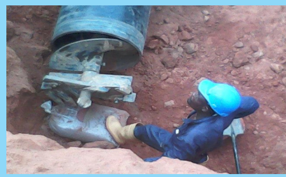
TRUST BORE PIPE PUSHING TO THE GROUND
