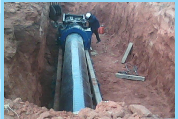
TRUST BORING PIPE IN PROGRESS AND CARRIER PIPE INSTALLATION
