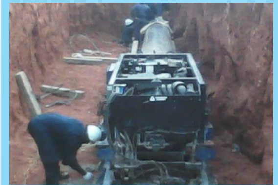
TRUST BORING PIPE IN PROGRESS
