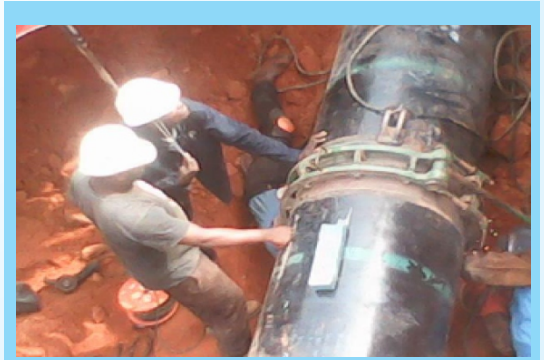
FITTING OF NEXT PIPE FOR TRUST BORING AND BEING INSPECTED BY QA/QC OFFICER
