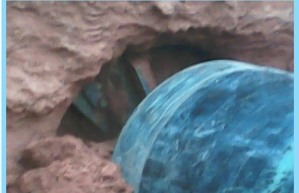
TRUST BORE PIPE ENTERING THE GROUND
