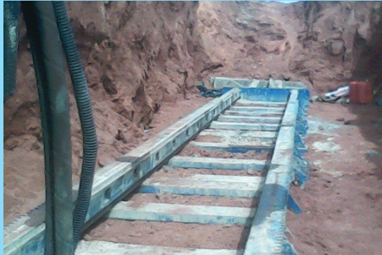
RAIL ALIGNMENT FOR AUGER BORING MACHINE TO MOVE ON
